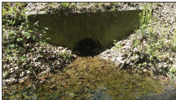
Figure 34 Culvert crossing, WCSWCD
