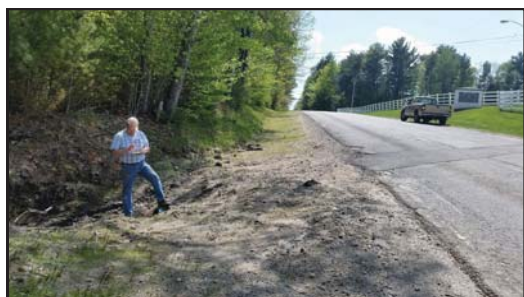
Figure 35 Culvert crossing, WCSWCD
