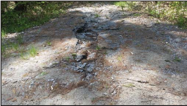
Figure 32 Driveway head-cut, WCSWCD
