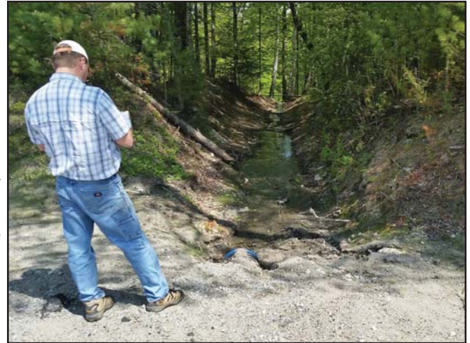
Figure 21 Inspection of a roadside culvert crossing, WCSWCD
