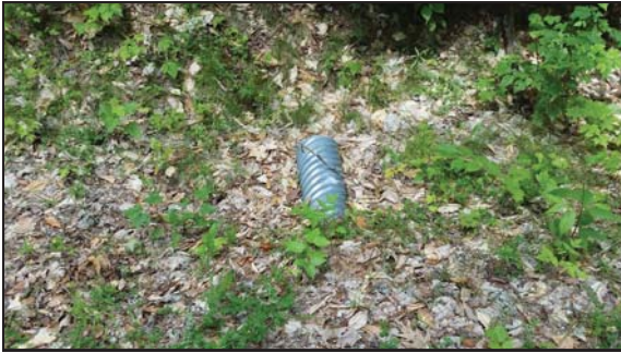
Figure 37 Culvert crossing, WCSWCD
