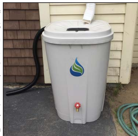
Figure 28 Rain Barrel, WCSWCD
